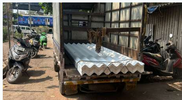
May-June 2026: Retrofitting activities underway in M-East & L wards
