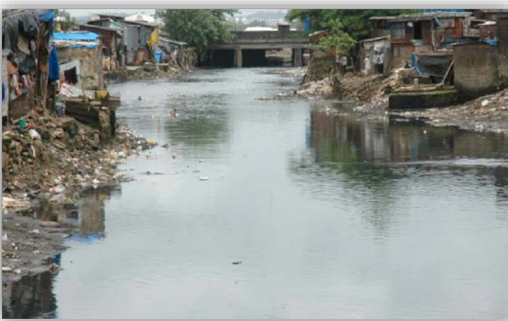
Near Krantinagar Bridge
