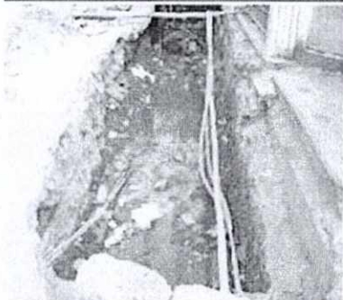
Storm water drains
