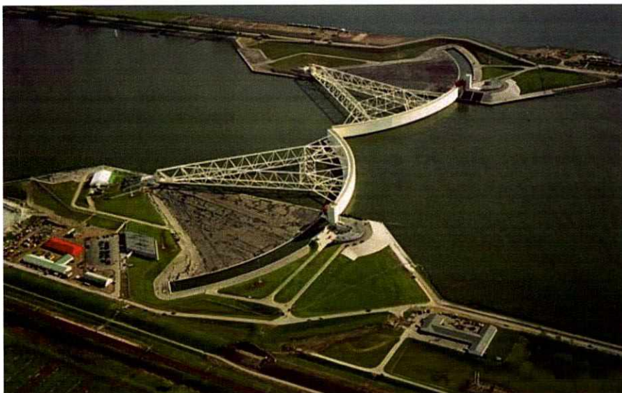
Figure 6.5: Maeslant Storm Surge Barrier Source: Official Site of Holland
