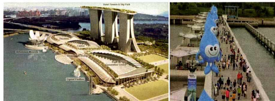
Figure 5.3: Singapore - Marina Bay Sands (left), Walkway on Marina Barrage Flood Gate Structure (right) Source: Marina Bay Sands, PUB
