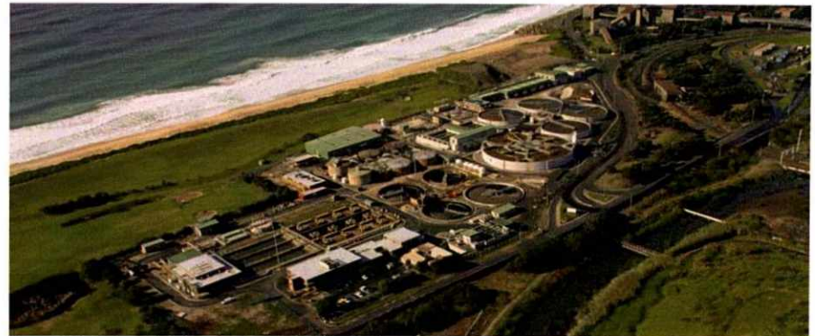
Figure 5.6: Sydney - Wollongong Recycled Water Plant Source: Sydney Water
