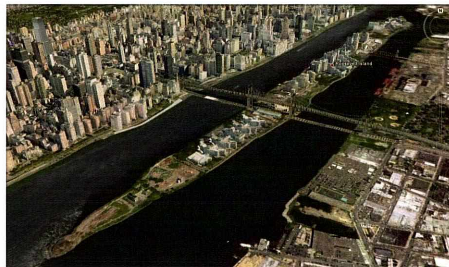
Figure 5.10: New York - Roosevelt Island Development Source: Google Earth
