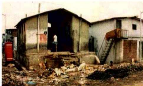
Figure 2.5: MMR - Conditions of Existing Public Toilet in Slum
