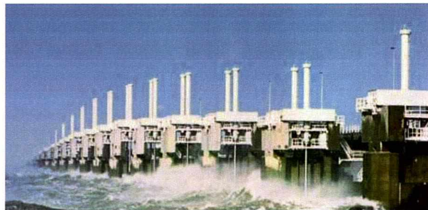
Figure 6.6: Eastern Scheldt Barrier Source: Official Site of Holland
